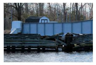
Figure 14: Damage to the southside fender of the North Landing Bridge.
