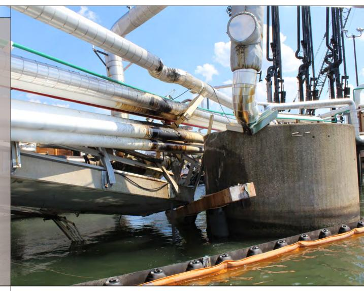
Figure 19: Damaged pipelines leading to loading arms on IMTT Bayonne Pier A.
